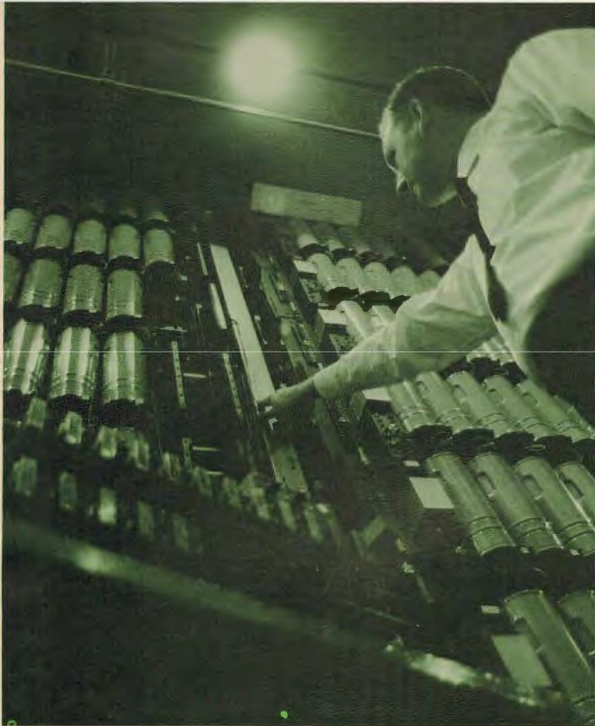
Special line identification equipment enables a telephone company switchman to identify the specific telephone from which an annoyance call was placed.
